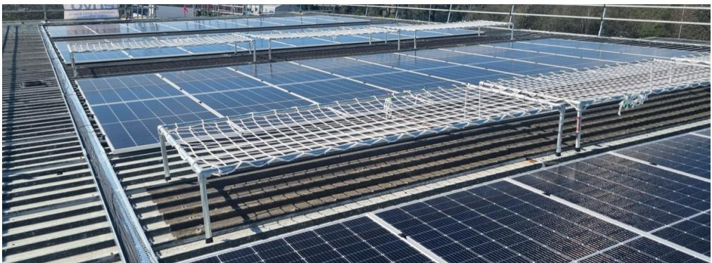
**Safety nets are the HSE's preferred method of fall arrest, reducing the need for a secondary method of rescue should a fall occur, whilst increasing the operatives chance of survival in the result of a fall.**
