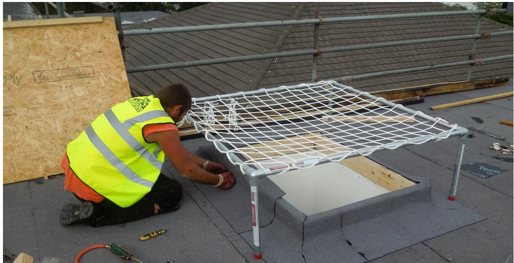
The Quadtube is equivalent in design performance to the Safetube but has the benefit of being supported on legs above a skylight aperture. This product is ideally suited to offer protection when carrying out localised repairs or replacing skylights. These are also ideal when applying liquid roof coverings, allowing virtually no interruption to the application process.
