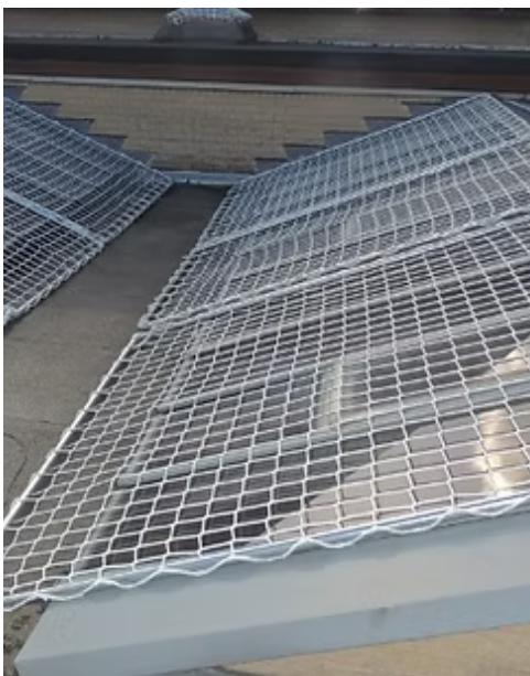
**If any doubt exists to the integrity of the skylight, the Safetube is placed over the fragile skylight without restricting access to the work area at any point. Where 'In Plane' roof skylights exist, these can also be protected with the Safetube and temporarily secured to the roof to prevent any movement during the works. Further reducing risk where internal slinging of a safety net is not always possible.**
