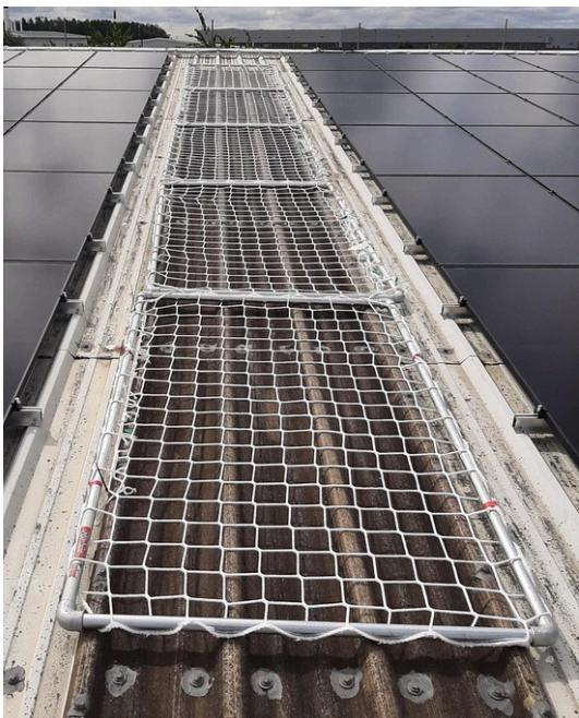
**Developed in the UK, Safetube and Quadtube Skylight Safety Nets are manufactured to BS/EN 1263/1, available in almost any size required, and can be installed in minutes. Each product can be reused on other high risk areas as works progress or can be left in-situ longer term for any future roof access that may be required, offering peace of mind for the building owner.**
