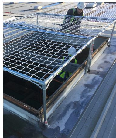
**No mechanical fixings are required into the roof structure as counterweights can be used or alternative temporary anti slip fixing points provided. HSE's Advisory Committee for Roofwork drop test demonstrates the integrity of the framed units under demanding conditions. No bulky handrail guards or temporary scaffolds are required around skylights, making them particularly useful on roofs where no existing or suitable fall arrest anchor system is installed.**
